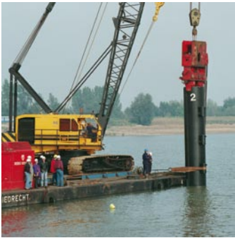
VIBRATING OF MOORING PILES
