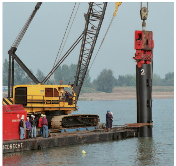
Vibrating mooring piles
