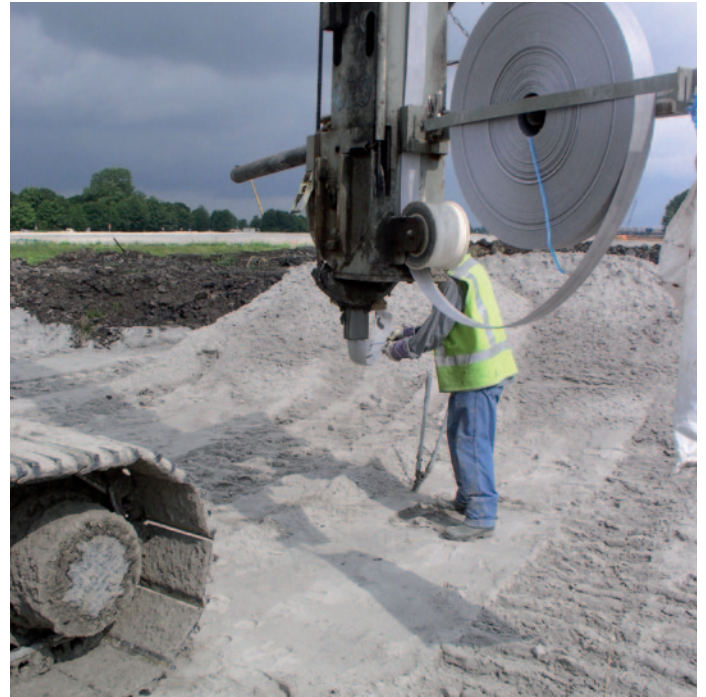
Installation of wick drains
