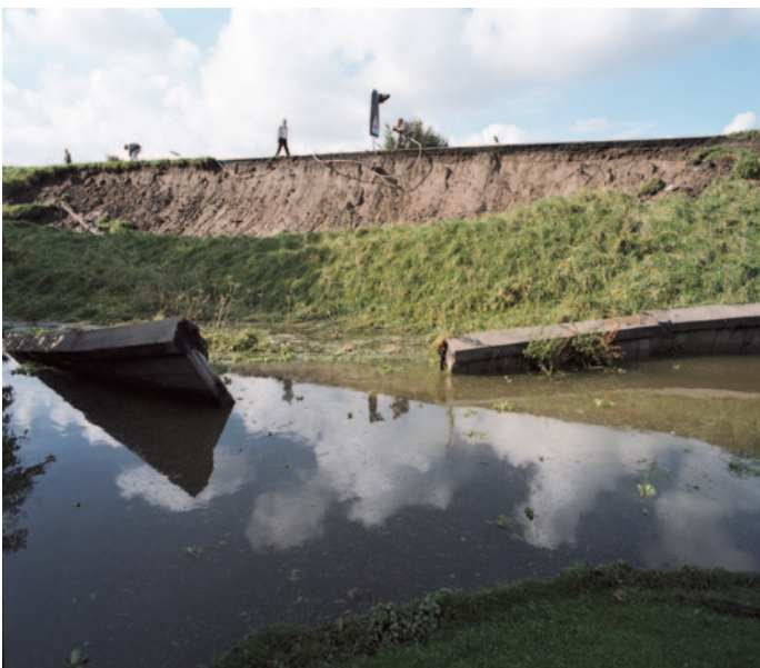
Embankment failure
