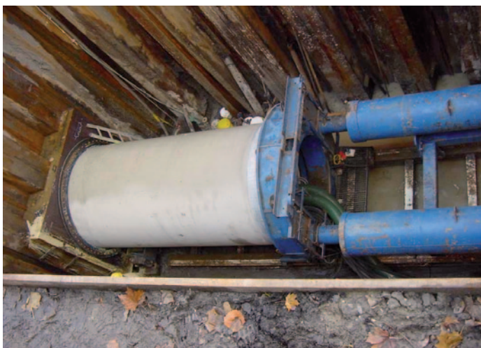
Hydraulic jacks in the start shaft
