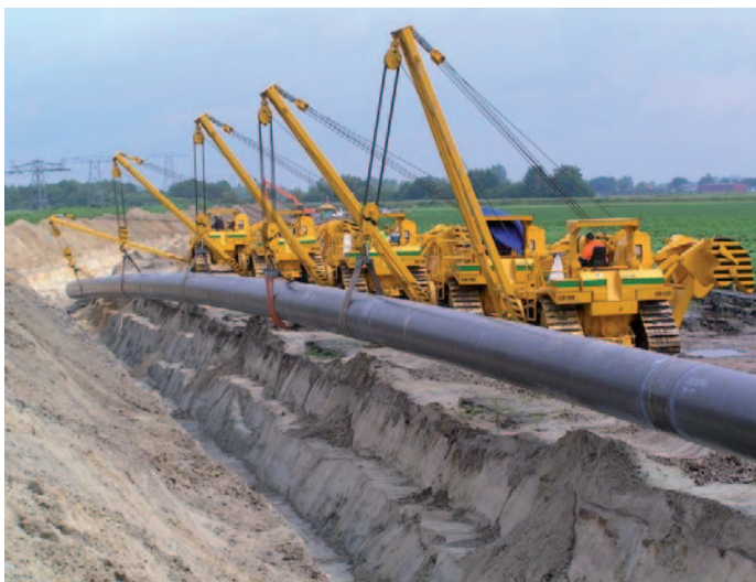
Installation of a pipeline into a trench
